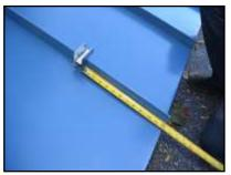
3. Set the first SnoBar Clamp onto the furthest left seam of the bar section at your 1st pencil mark. Hand tighten the set screws to the seam, making sure the clamp is centered and the bottom of clamp is pressed down tight to the top of the seam. The (2) holes in the bar receiver section of the SnoBar Clamp should be facing upslope when
